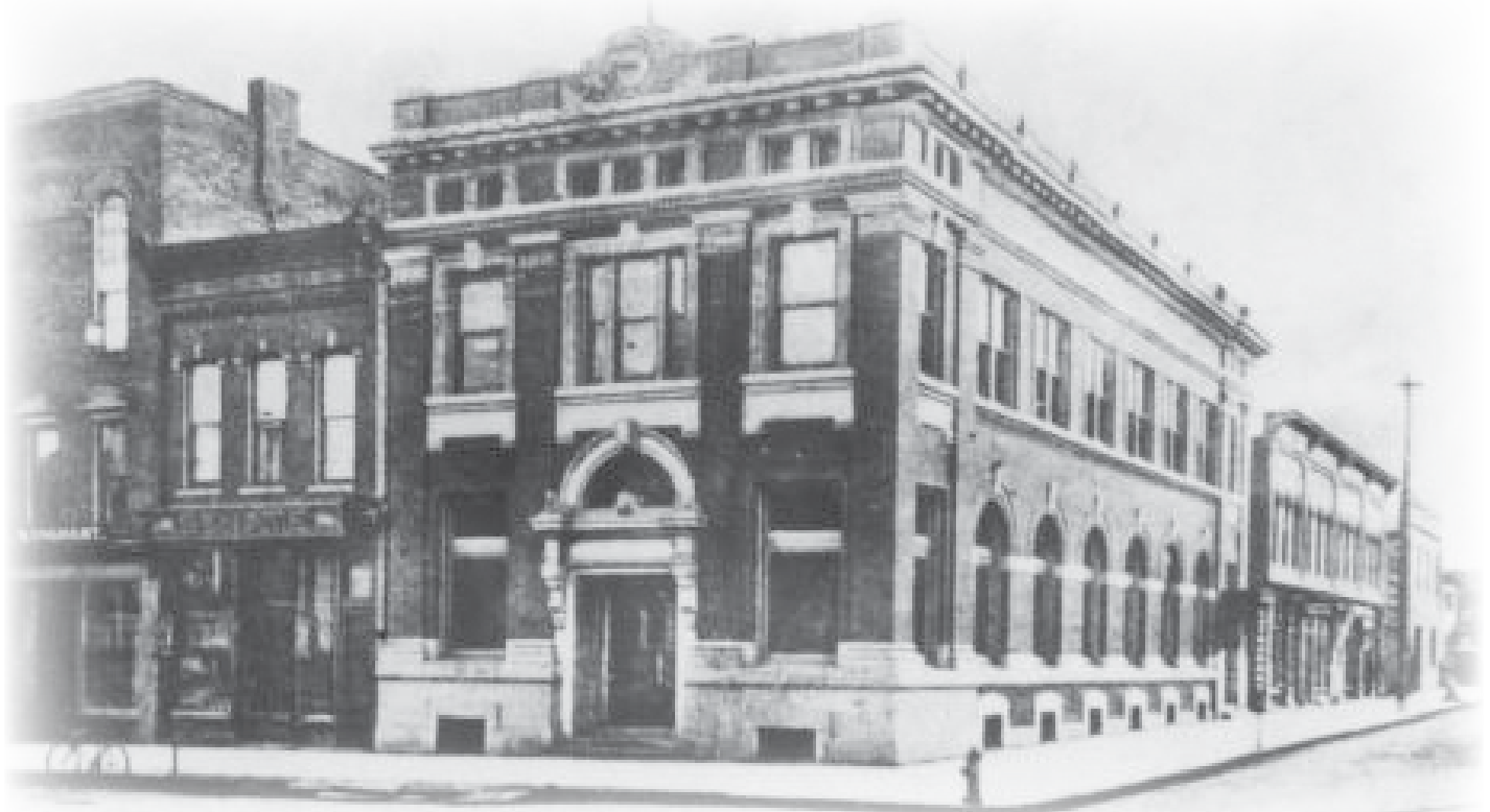
A photograph of the First National Bank of Ypsilanti building from 1909. This is how the building originally appeared, and how restoration work has returned it to its former glory.
