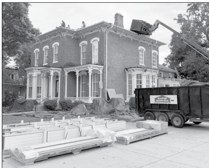
Work begins on replacing the museum roof, a much-needed renovation.
