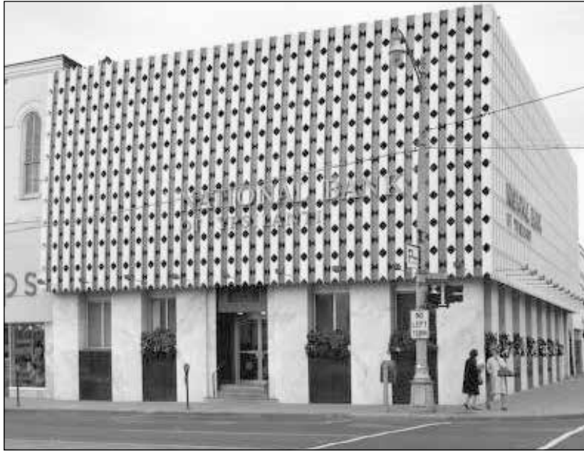
The building was given that "modern look" in about 1965 when the sides were covered with an aluminum "cheese grater." For this, the building was awarded the dubious honor of "Remuddling of the Month" from the Old House Journal in December 1982.
