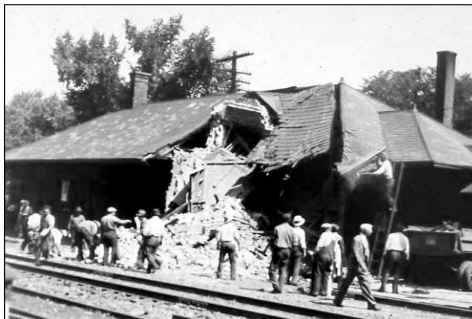
Damage to the depot from the train derailment of 1939.
