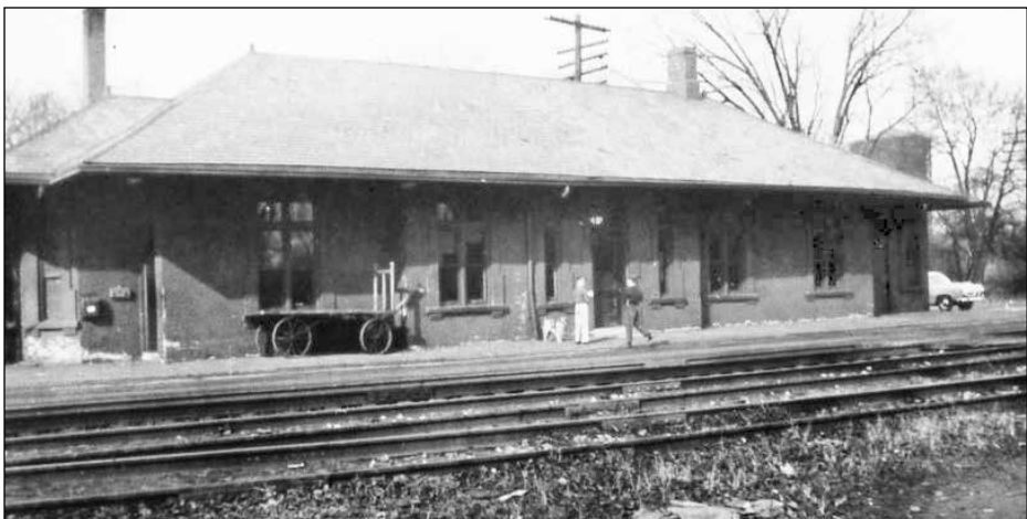
Depot after the repairs from the wreck of 1939.
