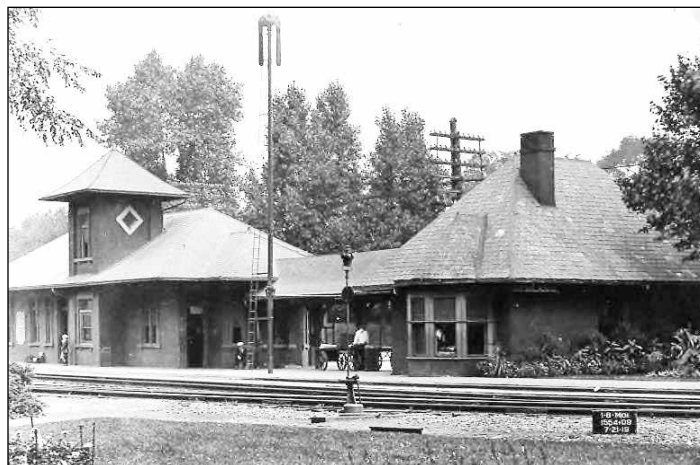
The depot as it appeared after the fire of 1910.
