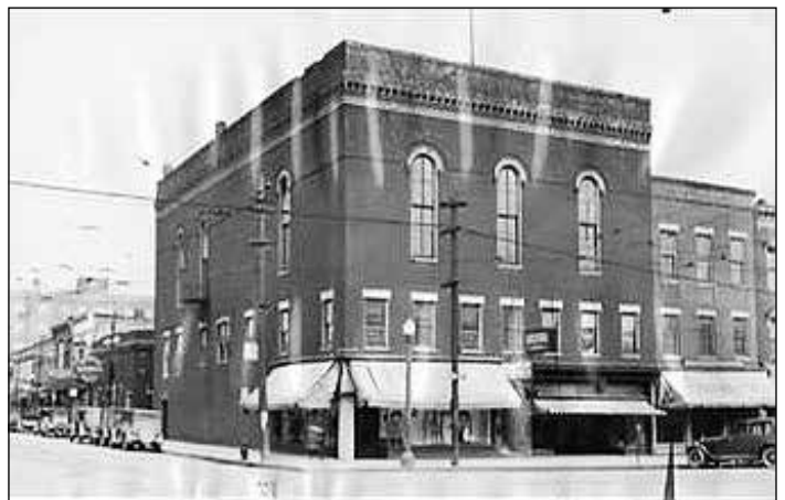
The three-story Hewitt Hall building at the northeast corner of Congress and Washington Streets was rebuilt after the fire.
