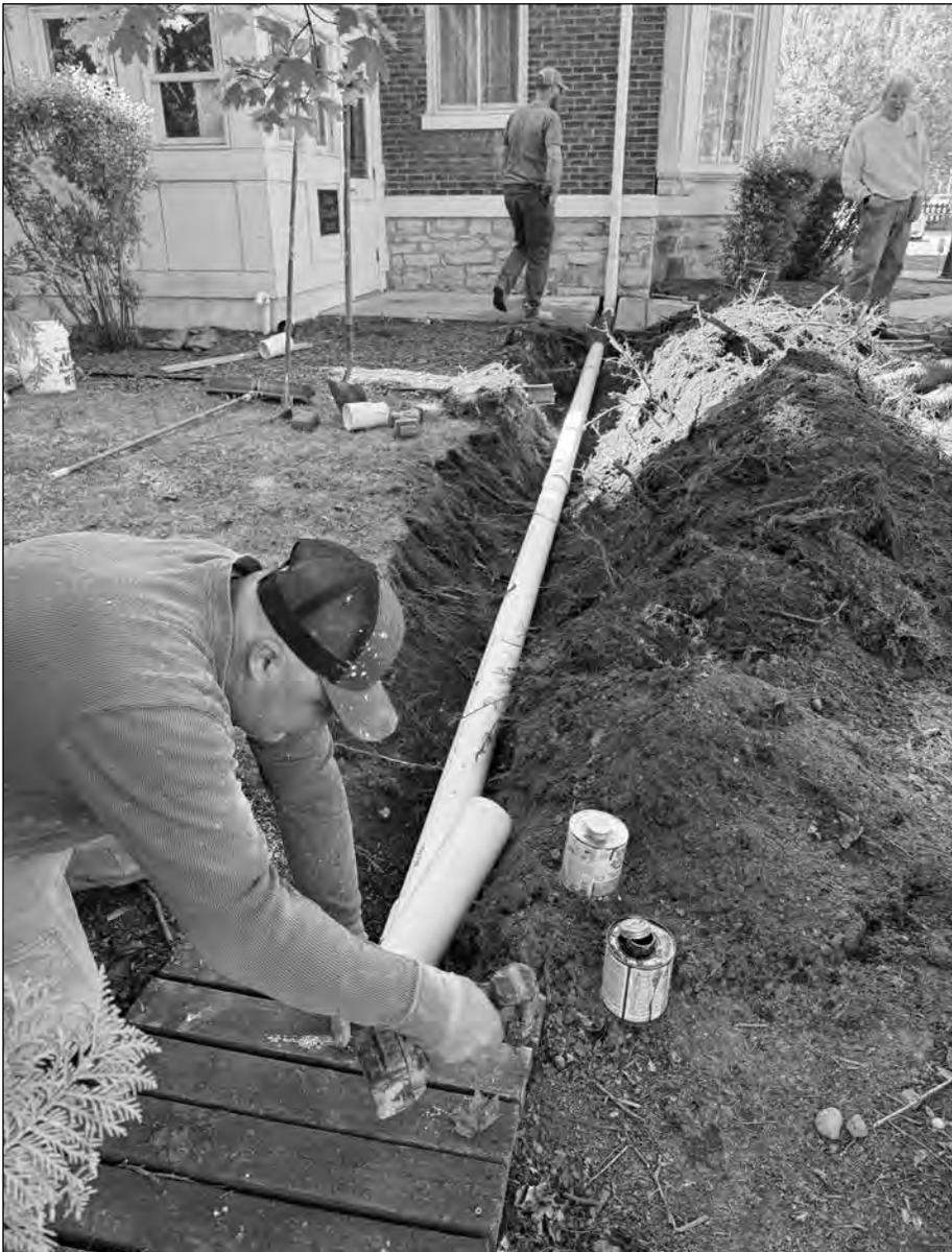
We completed our first 2025 maintenance project. An underground pipe was plugged with roots forcing water to out at the connection and leak into our basement archives. It is now fixed!
