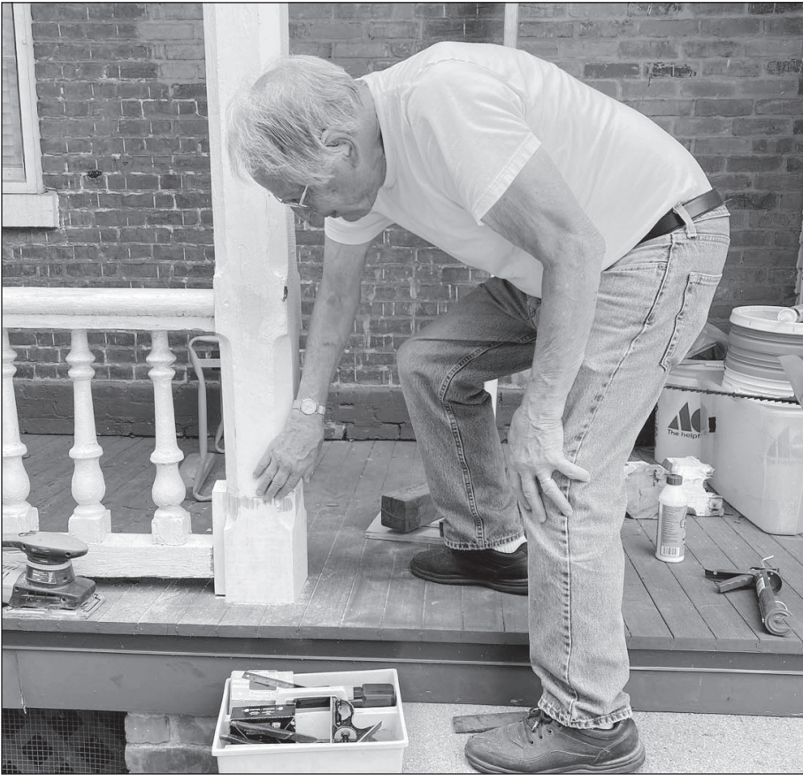
Jerry Jennings repairing the back porch on the Museum.
