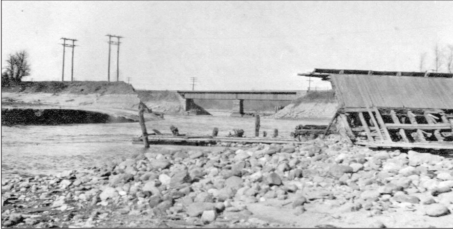
Superior Dam after the flood of 1918.
