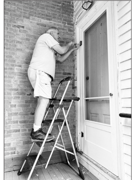
Volunteer John Harrington installs a restored back porch storm door.
