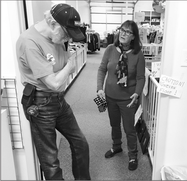
Jim Aulenbacher discusses uneven floor with Debbie White.
