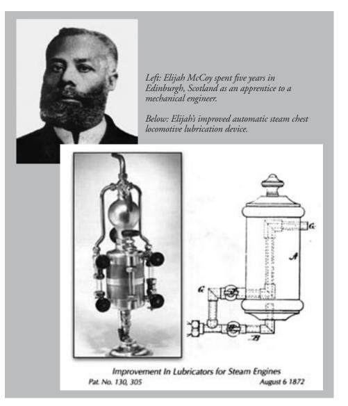
this reality significantly slowed rail travel. Elijah soon realized the need for a device to provide oil directly into a railroad engine and he set out to create one.
