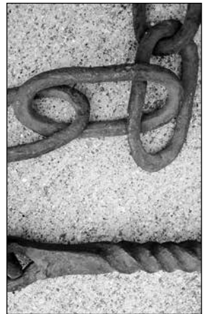
Detail of the individually forged links connected to the grip bar which has been twisted.
